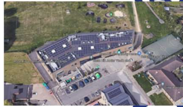
Rose Hill Community Centre – solar array
