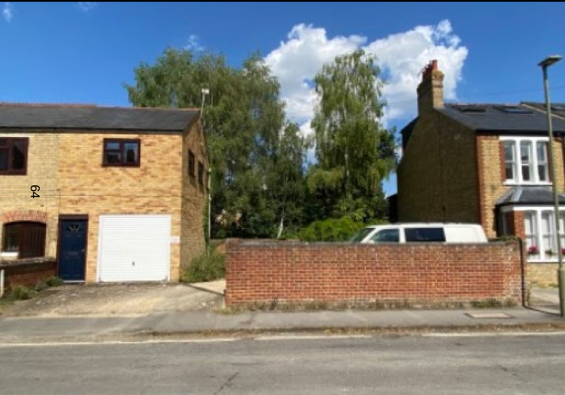
View of the southern part of the application site, facing Stratfield Road)
