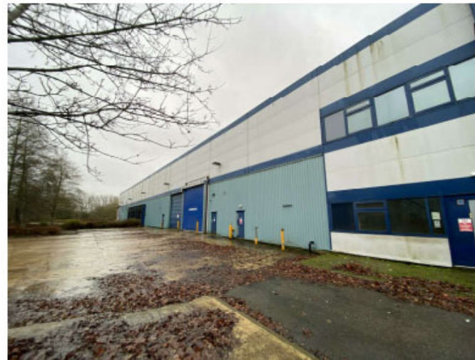
EAST ELEVATION LOOKING SOUTH
