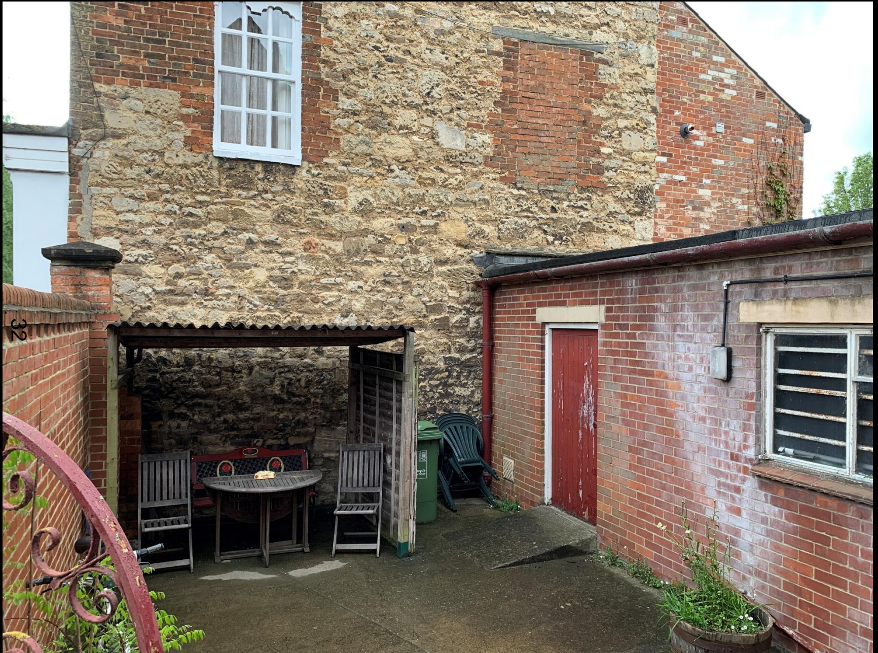
View of the rear yard of 1 North Street
