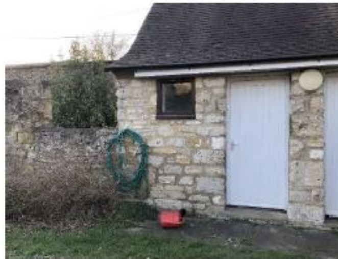
d. Exterior of utility showing example of the modern alterations and poor quality repointing to the stonework evident throughout the building.
