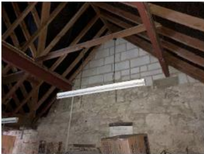
c. Interior of garage showing modern blockwork alterations to create the gable of the stables and new roof structure
