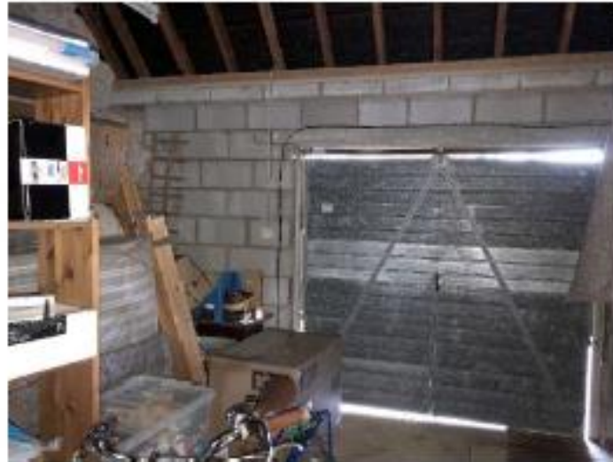
b. Interior of garage showing modern blockwork and new roof
