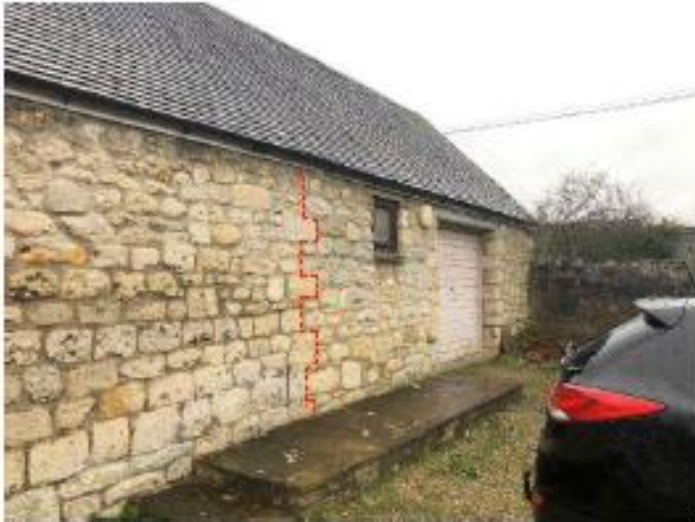
a. 1970s alterations clearly visible around creating of opening for garage door and removal of original gable and break in building line
