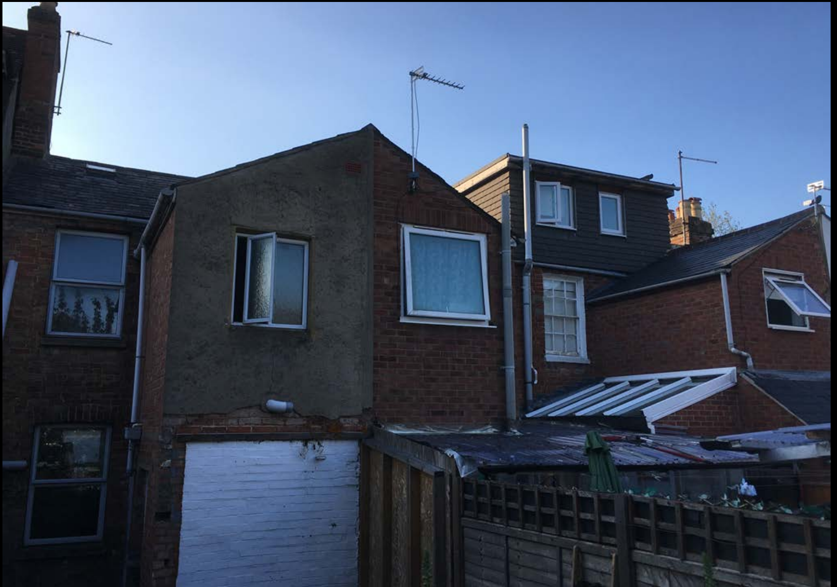
View of the rear of the site (3)
