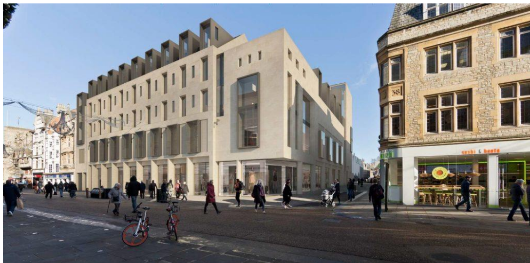
Image 1: Northgate House upon completion
