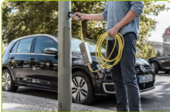
Simple Socket & Smart Cable - Lamp Column Charging Point
