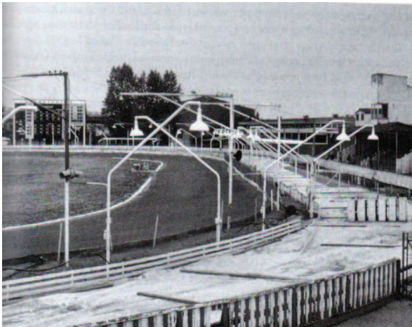
Fig3: original floodlighting (c1939) at Oxford Stadium. These lights (now replaced) were both a projection of the modernism of the stadium -a significant aspect of the servicing of 'pleasure buildings' more broadly- and a crucial aspect of the 'drama' of a racing event. The stadium was darkened before a race and a switch (still present) would swing the lights onto either the dog or speedways track depending on the event. An aspect of this is visible on the image with some lights focused on the dog track in the foreground and others on the speedways track adjacent to the central green. The southern grandstand (since rebuilt) is also visible on the right with the tote building across the central green on the far left corner.
