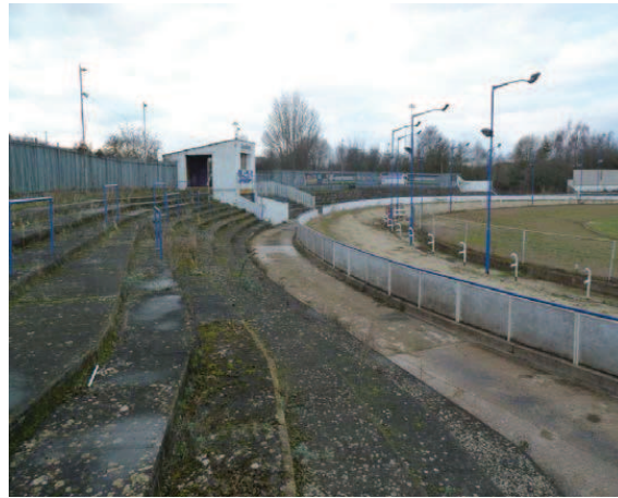
Fig 4: The concrete western terraces (built c 1939) are in many ways exemplary of their time both in their design and materiality (i.e. form). Their location in quite close proximity to the dog tracks catered to the 'modern desires' of their audiences who increasingly sought more heightened sensorial stimulation through greater contact with the 'main action'. Their curving design following the general line of the track enable spectators to view the unfolding of a race from start to finish without the need for binoculars as was often the case with other sports such as horse racing. Their material construction – consisting primarily of large expanses of moulded concrete - embody the modernist movement's preoccupation with ephemeral as well as catering to the need for expedience that was generally necessitated in the construction of pleasure buildings.
