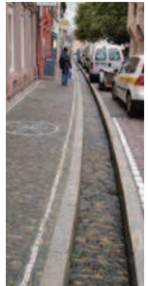
Water management rill in streetscape
