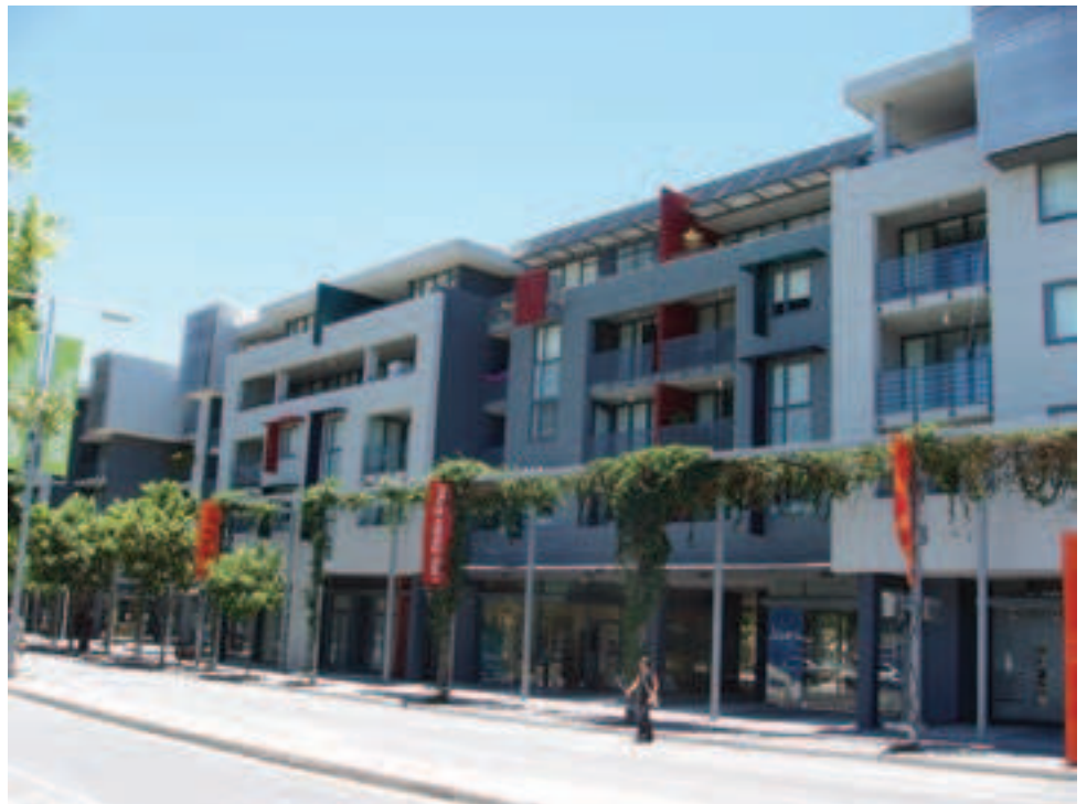
Mixed use buildings with strong street frontage, especially at Oxpens Road
