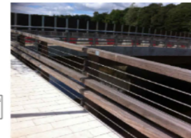
Image 2: Bridge parapet (alternative) - Sarum Hardwood N2 Parapet, or similar
