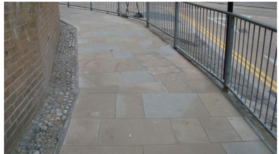
Cobbles in relatively poor condition and modern paving on the corner of Paradise Street and Castle Street. The galvanised steel railings do not contribute positively to the character of the conservation area
