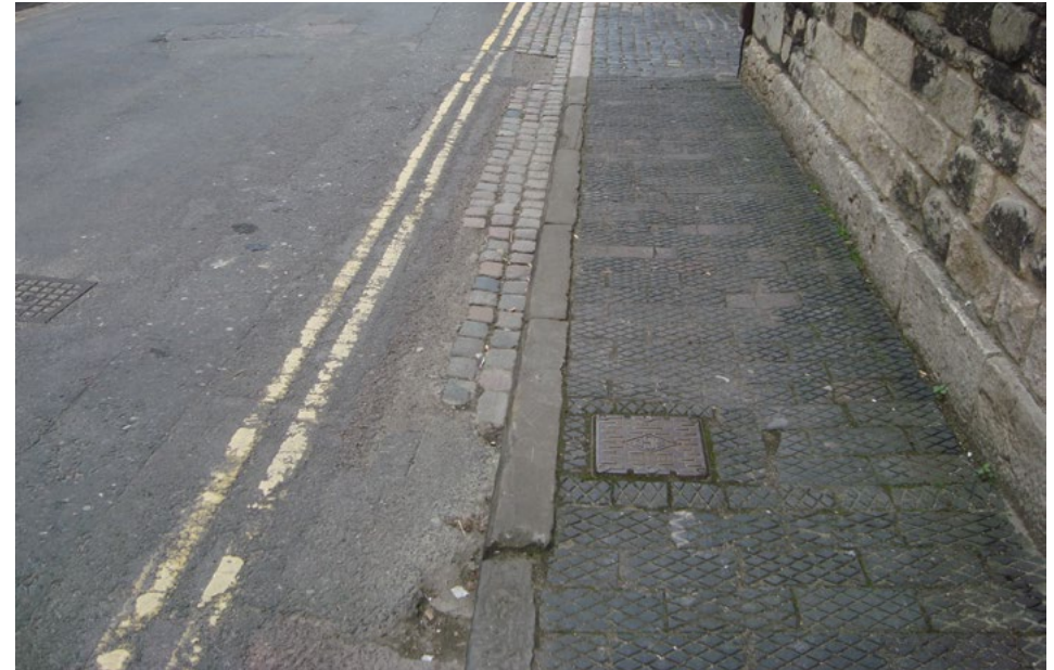
Blue clay pavers and granite sett gutters on Tidmarsh Lane
