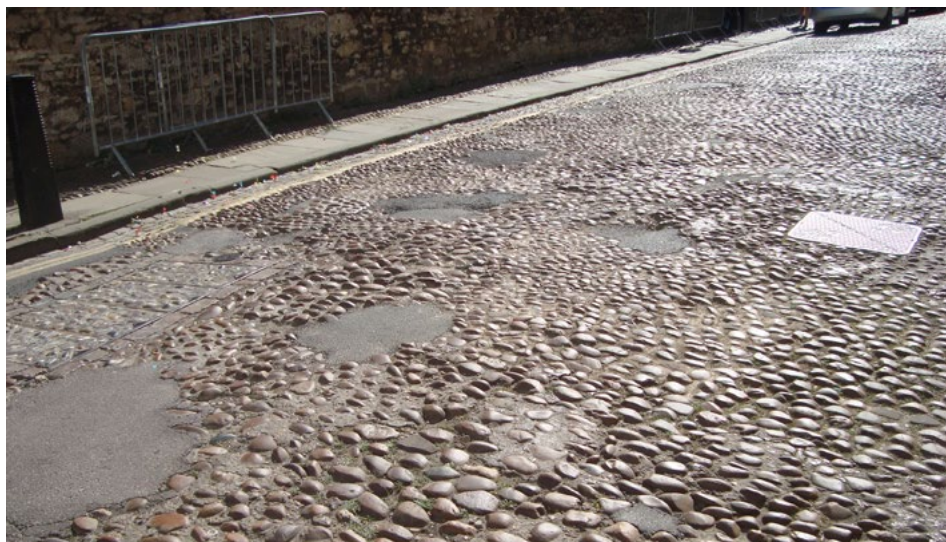
The historic street surface of Merton Street is marred by missing cobbles and poor quality repairs
