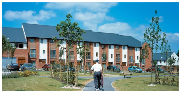
Affordable housing at Oakridge Village, Basingstoke (HTA Architects/@TimCrocker05)
