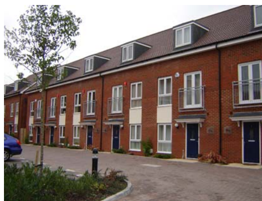
Affordable Housing at Rivermead Park, Oxford
