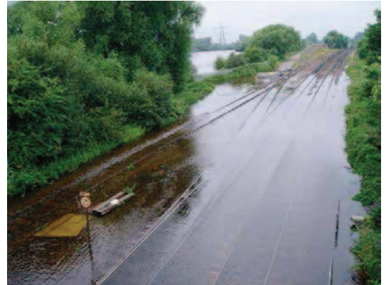
Impact of flooding on transport links – flooding of the railway line north of Old Abingdon Road. July 2013.
